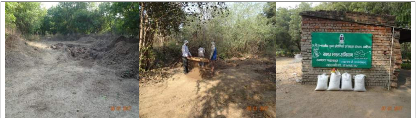
Organic Waste Treatment,
